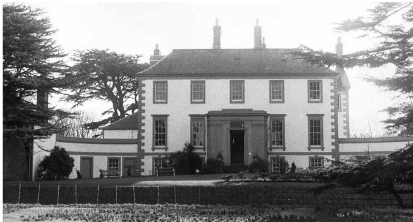
Below: Rozelle House, Alloway with post 1837 side extensions.
